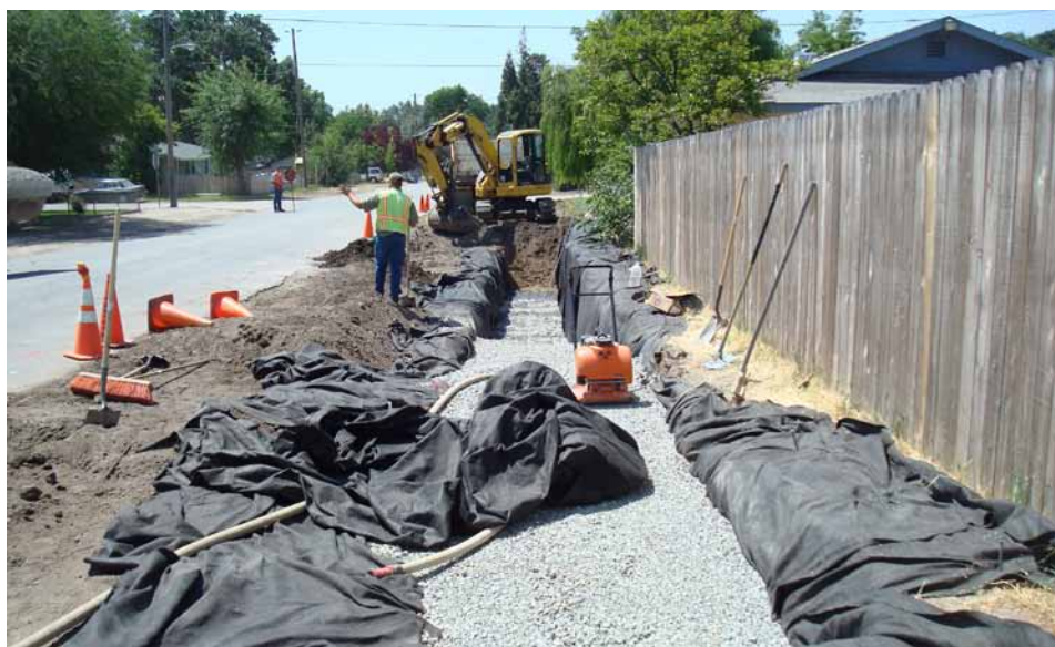
Installation of infiltration basins along the edge of a roadway.
