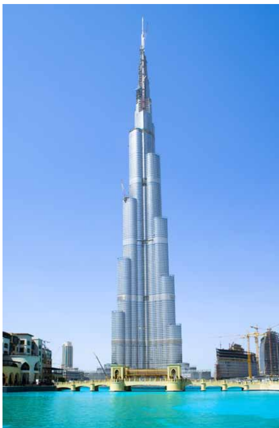
Burj Khalifa in Dubai, UAE, the world's tallest building.
