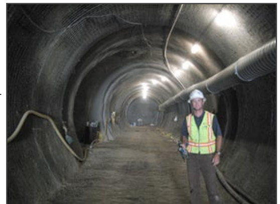
Earth Systems' Judd King inspecting wine cave construction
