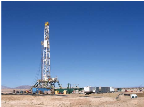
Geothermal exploration well being drilled in Imperial County, California.
