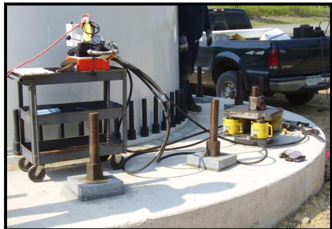
From Finite Element Analyses to Anchor Tensioning & Load Testing to Verify Performance
